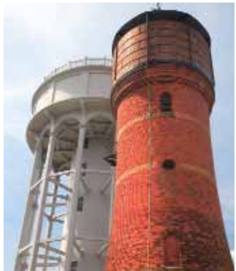
Rockwell Green Towers restoration, Wellington, UK
