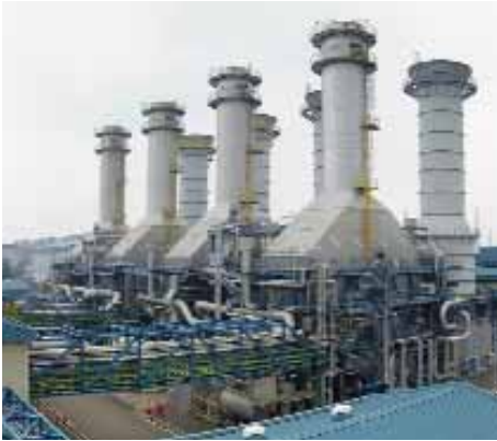
YTL's Paka Power Plant – a gas-fired power station is one of three plants that generate some 2,500MW of electricity for the state of Terengganu
